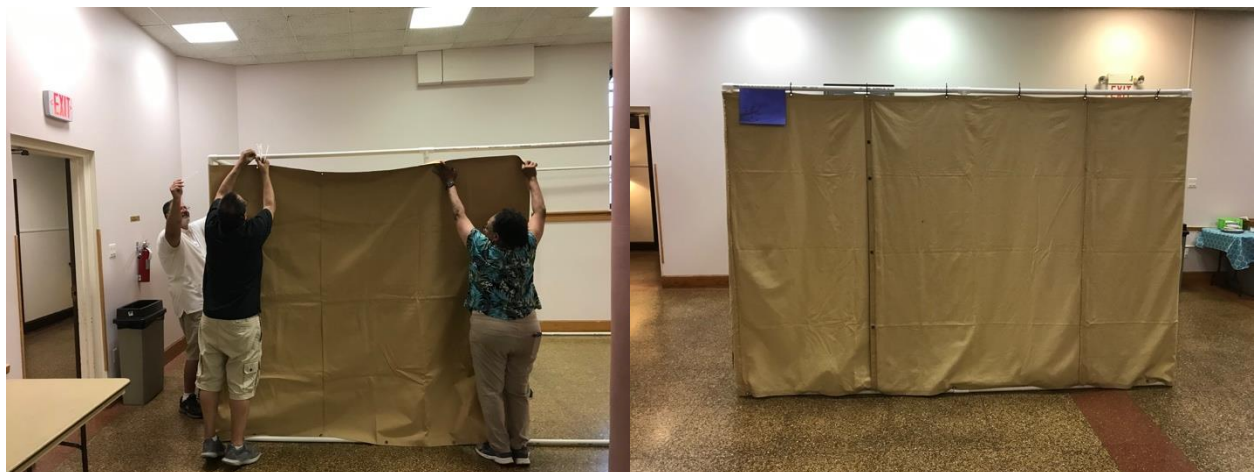
Construction of sleeping quarters
